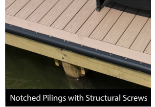
Notched Pilings with Structural Screws
